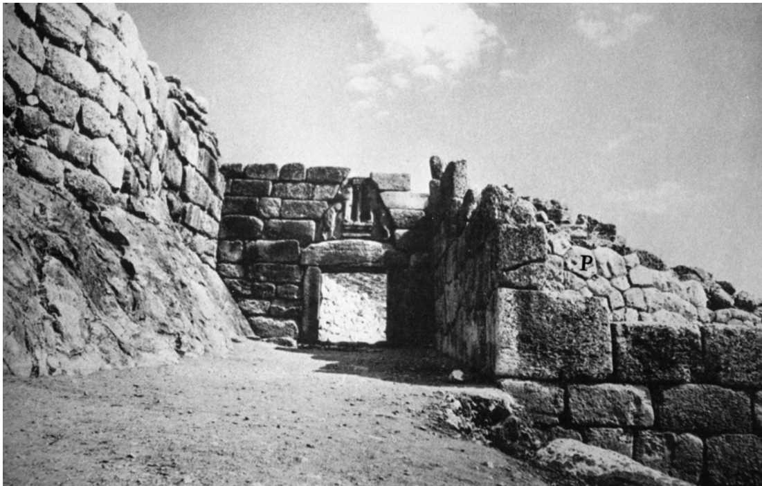
Figure 11. The city wall of Mycenae includes in its lower part and as its foundation a natural fault scarp dipping here at 60 deg. or so. Even a very modest earthquake on this fault would cause the wall to tumble, and render it ineffective for defense against attack (after Mylonas, 1996: fig. 11).
