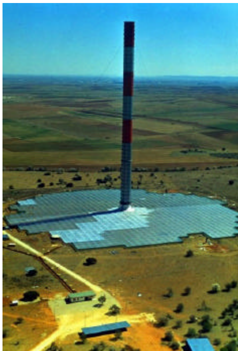
4-5: Prototype Solar Chimney in Spain
