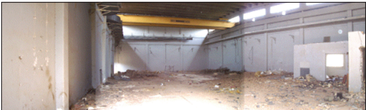
Figure 8. Al Hamath facility.
