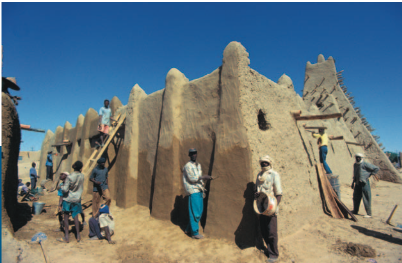
The restoration of the ancient mosques of Timbuktu was carried out by local craftsmen using traditional practices.
