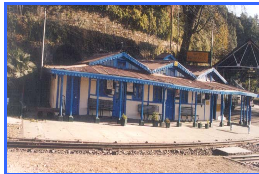
Kalka-Shimla Rail Line
