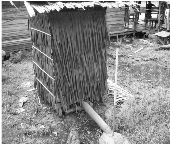
Locally innovated toilet model in flood prone areas and in places with high water table. Sambas West Kalimantan.
