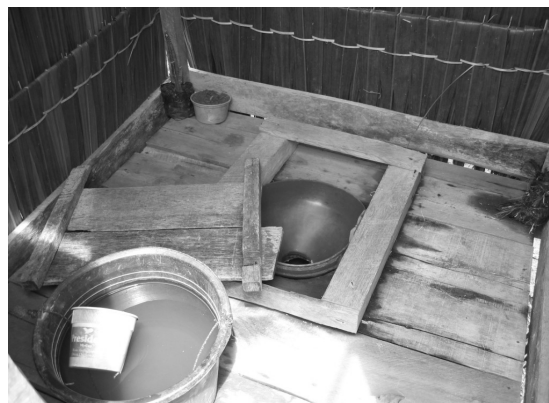
Using plastic funnel as toilet pan: an immediate measure to declare the village free from open defecation, South Sumatra, Indonesia.
