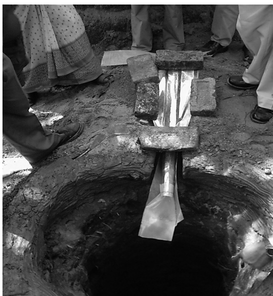
Tin sheet, old plastic bottles and plastic sheets are used to construct toilets.*
