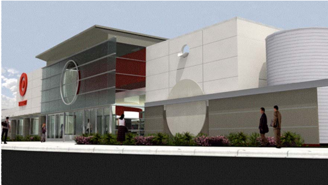
Rendering of the Allen Park, Michigan Target store, which opened in October 2005. Rainwater will be captured using a rooftop cistern (shown on the right).
