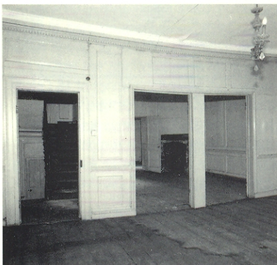
BELOW: Benjamin Franklin's Parlour, showing (right) the work necessary to counteract the sagging
