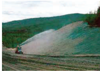
Figure 88: Hydroseeding a large-cut slope. This is the ideal area and use for a hydroseeder.
