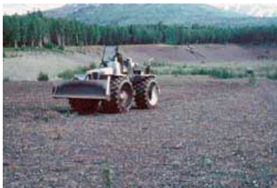
Figure 102: A landfill compacter being used to loosen and imprint the surface of an old gravel pit.
