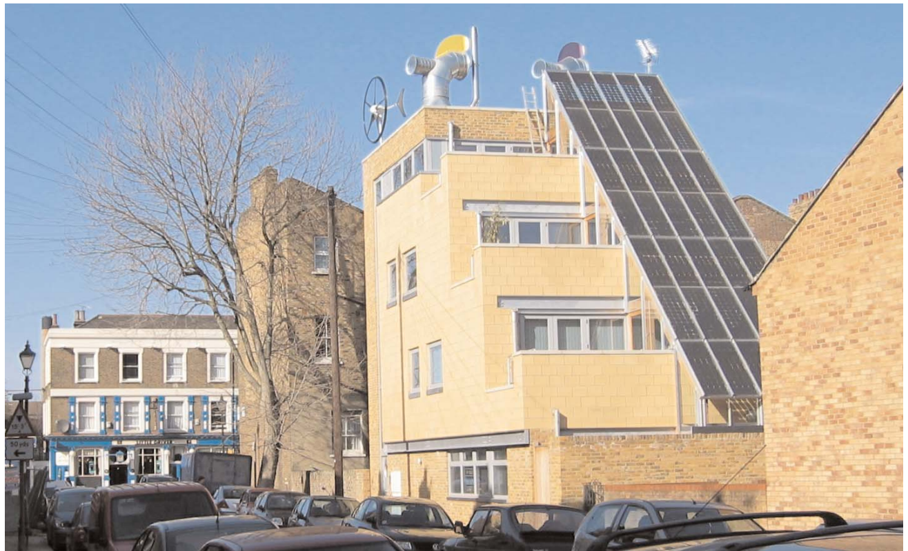
Above: BowZED's PV laminate glazed sunspaces
