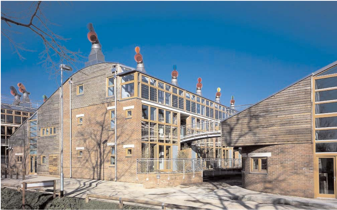
Above: The gable end treatment of BedZED introduces a new urban typology using local traditional materials.
