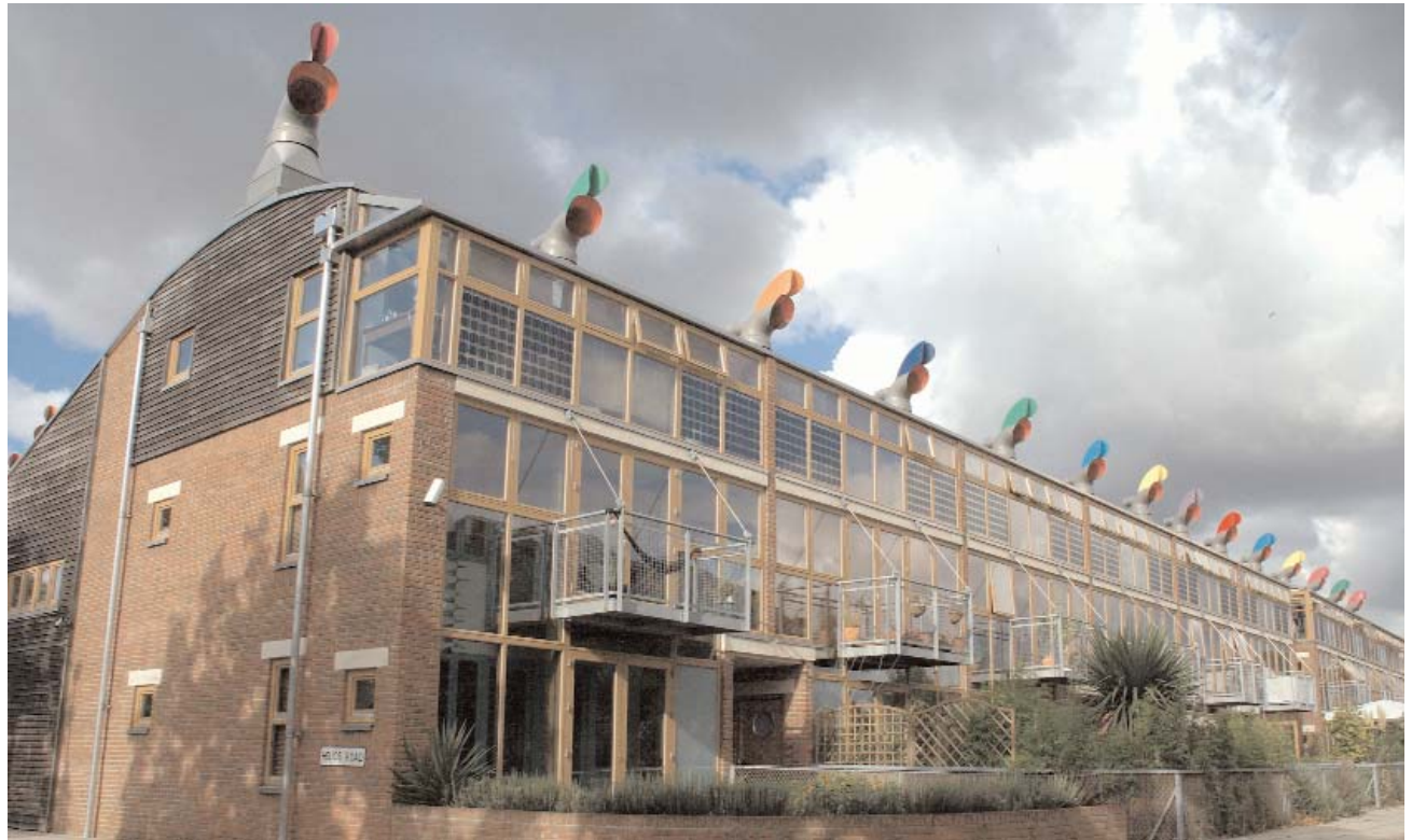
Above: BedZED as it looks today after 4 years of occupation. The pallet of natural materials was chosen to age gracefully with minimal maintenance.
