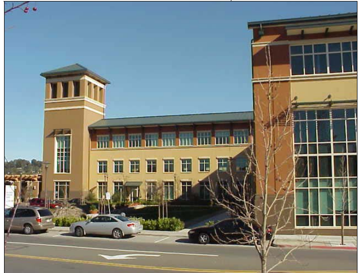
The San Rafael Corporate Center, a Class A office development, is a redevelopment of a Brownfield site in Downtown.
