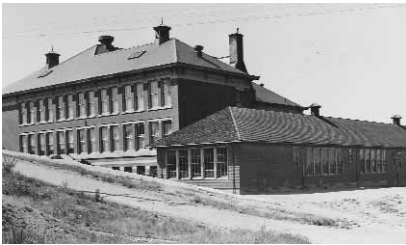
Jefferson and Jefferson Annex, ca. 1945 SPSA 238-254
