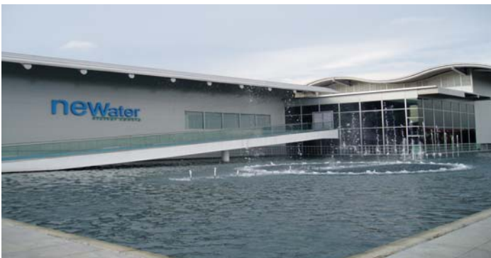
NEWater visitor center, Bedok, Singapore.
