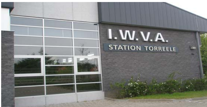
Torreele water reclamation plant, Wulpen, Belgium.
