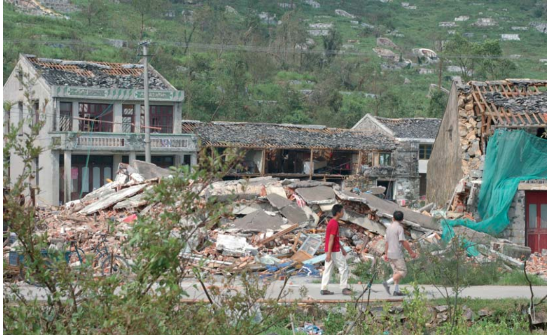
FIGURE 3: EXTENSIVE DAMAGE IN HONGLINGXIA VILLAGE NEAR THE TOWN OF JINXIANG
