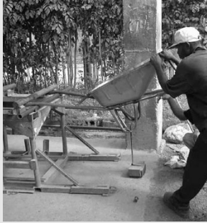
Figure 20: Cintrage du tube principal
