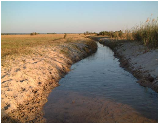
Figure 14: Hand-dug dyke, built at turn of twentieth century, recently renovated but not yet put to good use in cultivation (Old Limulunga district, Western Zambia, April 2005).
