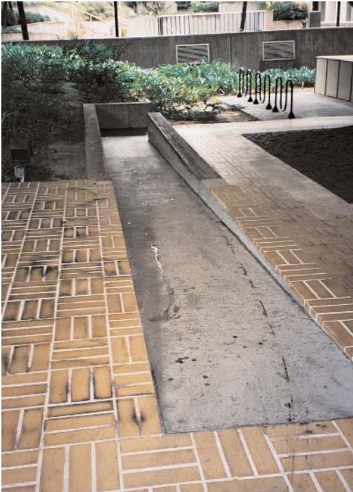
Figure 18: The accessible ramp at the plaza an early use of this type of entry feature.
