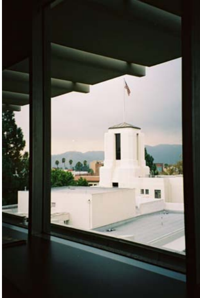
Figure 1: View of the City Hall tower to the west from Cafeteria of the Municipal Services Building.
