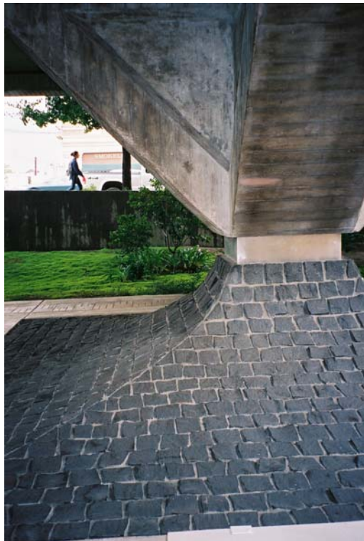
Figure 4: A detail of the piloti.
