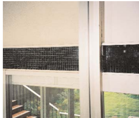
Figure 6: Tile frieze is present at both the interior and exterior of the building.
