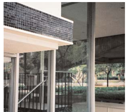
Figure 7: Tile frieze at exterior corner
