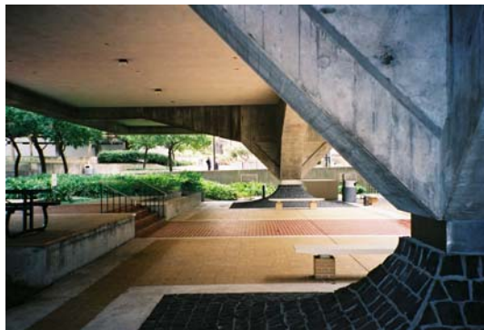
Figure 3: The plaza and piloti faced with rough granite pavers.
