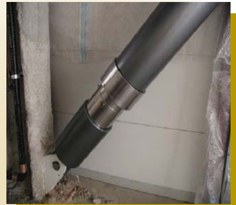
Figure 2: Fluid Viscous Damper
