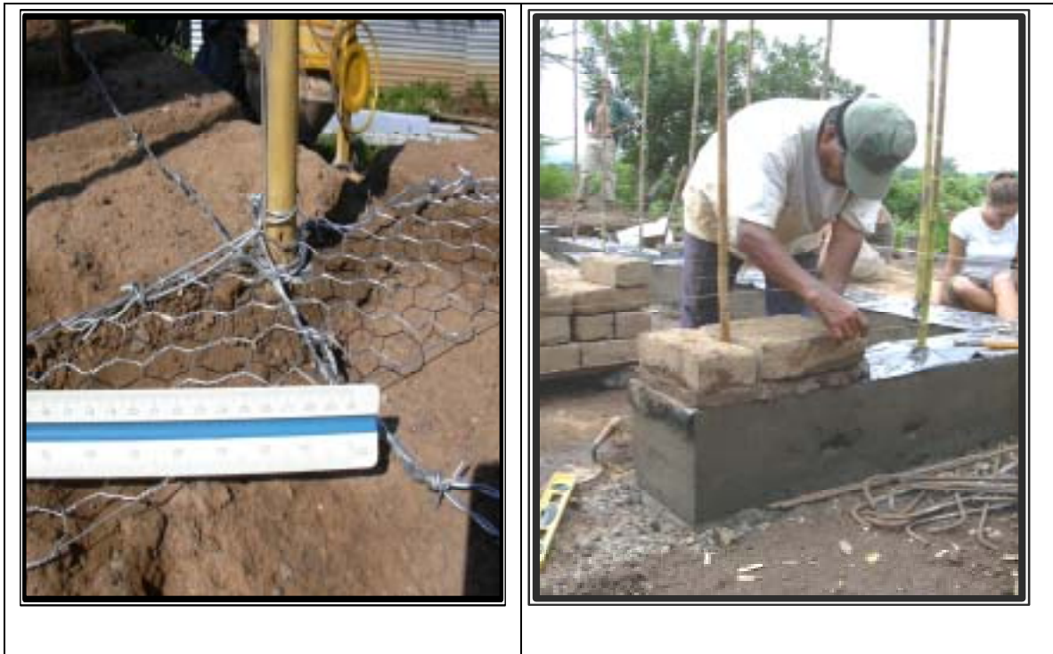
Figure 12 – Construction of Cane Reinforcement In El Salvador (Dowling 2002)
