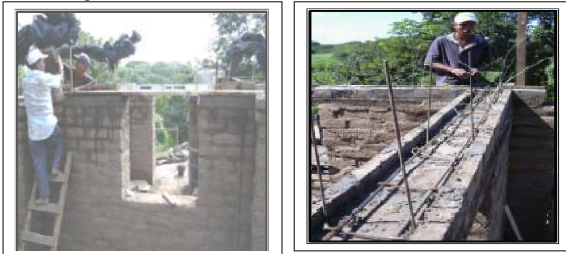
Figure 16- Reinforced Concrete Lintel Ring Beam Construction in El Salvador (Dowling 2002)
