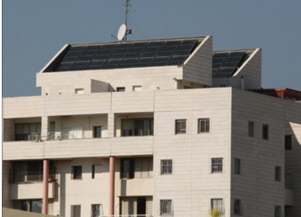
One way in which solar collectors can be architecturally integrated into apartment blocks.
