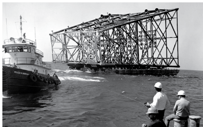
The steel jacket for the Barracouta platform was towed to the offshore field in the Bass Strait in 1967.
