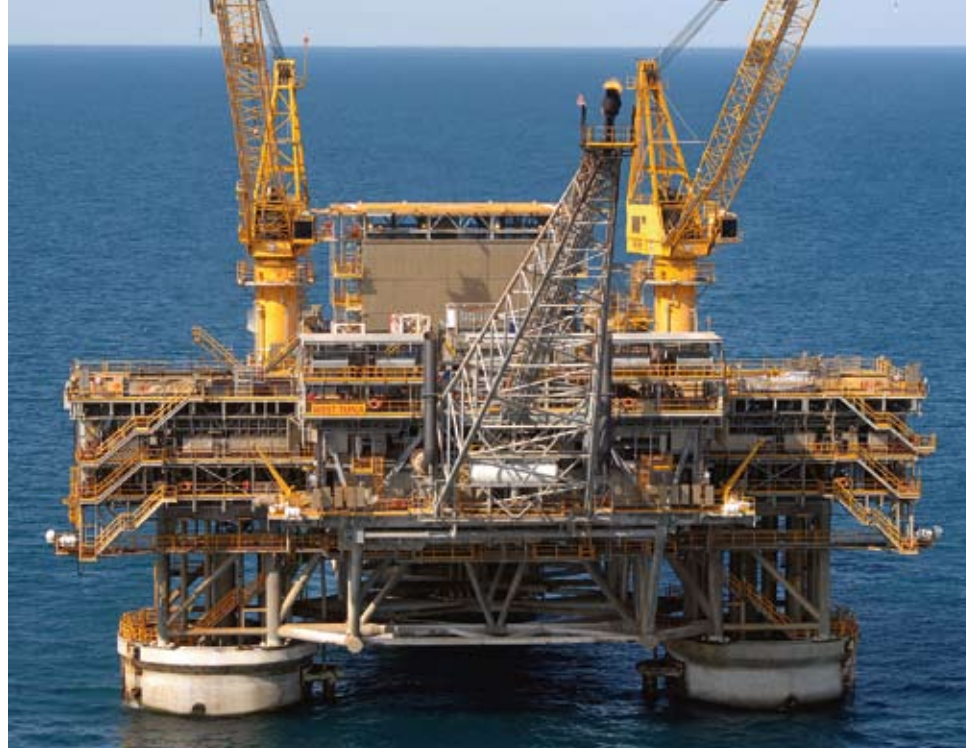
New oil and gas projects continue with the combined $2.1 billion Kipper/Tuna and Turrum projects, expected to begin production in 2011. The Kipper field will be developed by the installation of a number of subsea wells, tied back to West Tuna Platform (pictured) and piped to existing infrastructure onshore.
