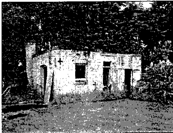
Brick outbuilding (DPAL, 2005).
