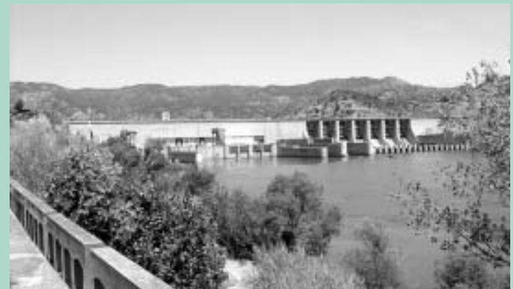
The Riba Roja dam on the Ebro River. WWF-Spain
