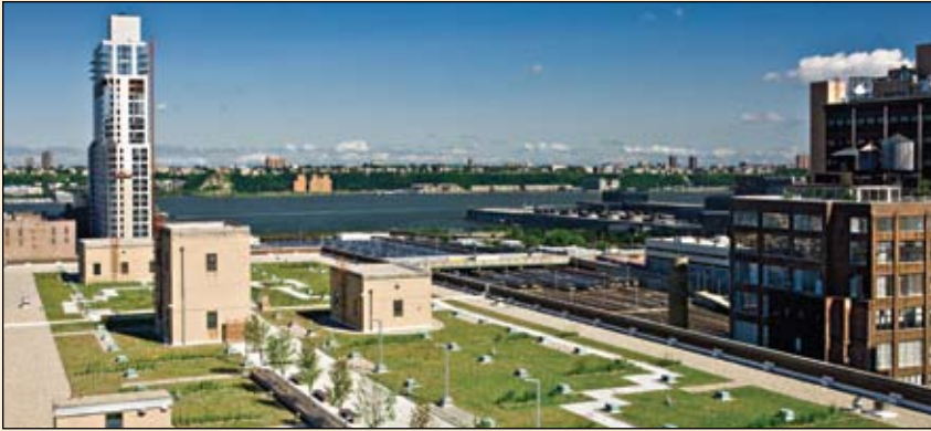
The Postal Service has the largest green roof in New York City.
