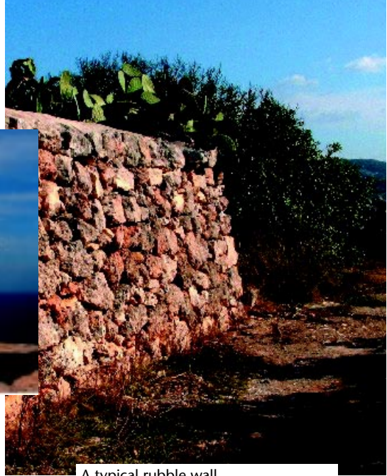
A typical rubble wall
