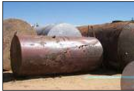
Old underground storage tanks.
