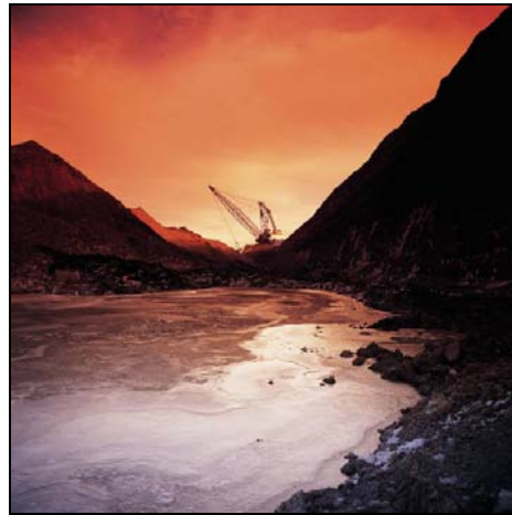
A construction site near water.
