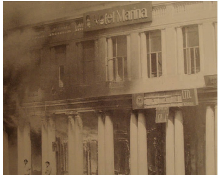
Hotel Marina on fire, Connaught Place, commercial centre of New Delhi. Photo by Ashok Vahie
