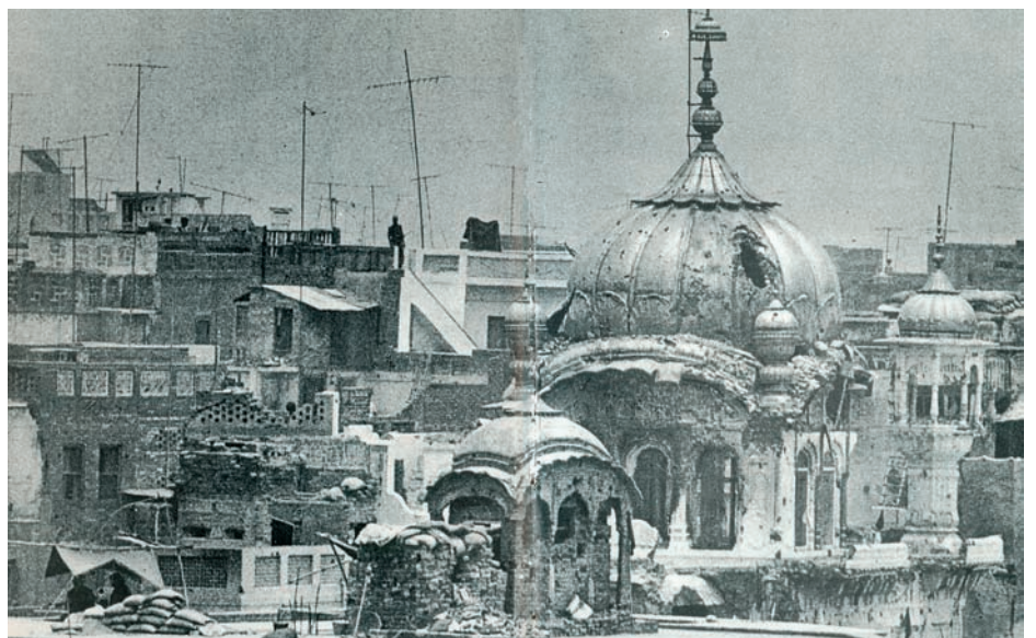
The damage to the Akal Takht's golden dome. Courtesy of India Today
