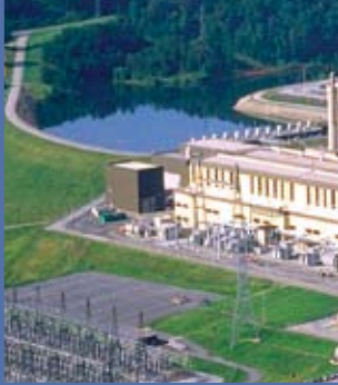
Oconee Nuclear Power Plant, Seneca, South Carolina.
