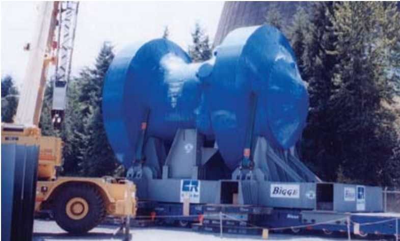
Reactor vessel being transported during decommissioning of the Trojan Nuclear Power Plant.
