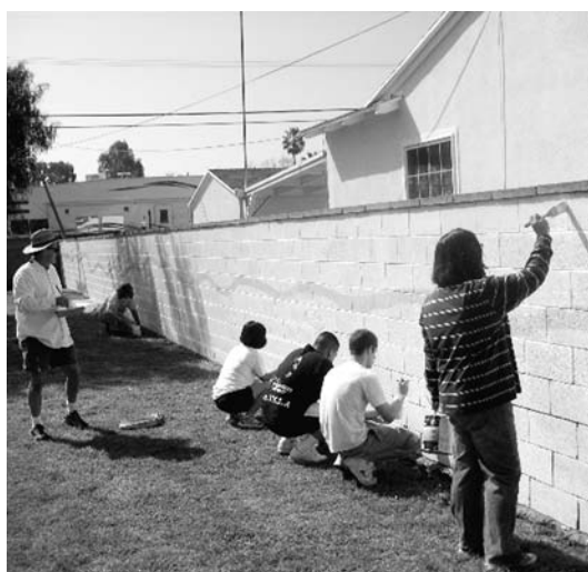
A group of volunteers prep the wall and layout the underlying design.
