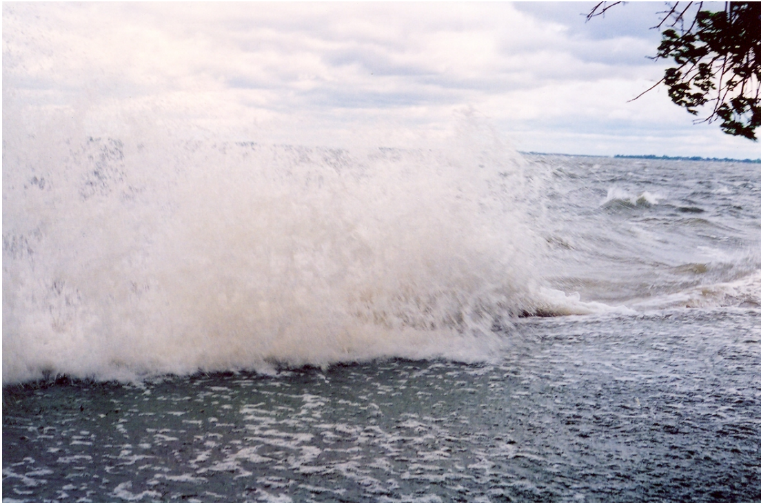
Figure 9. Flood level waves deflected by submerged steel wall.
