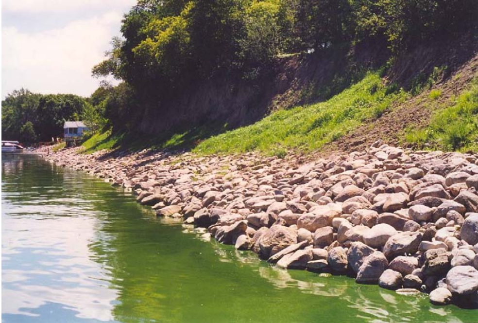
Figure 7. Two years after stabilization using geotextile fabric and field rock.
