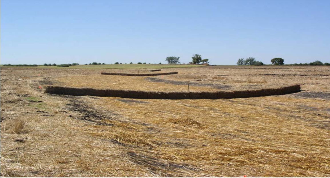
Figure 14. New waterway with erosion control in place.
