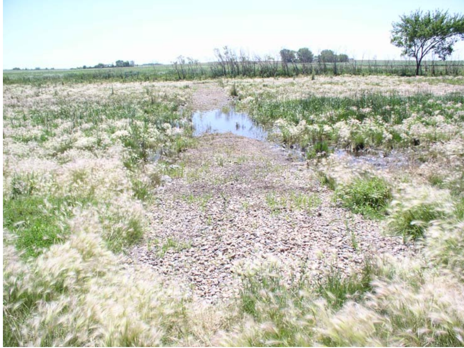
Figure 10. Rock crossing of small stream in flood plain.
