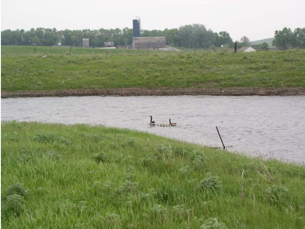
Figure 16. Small pond constructed to trap sediment from upstream cropland.
