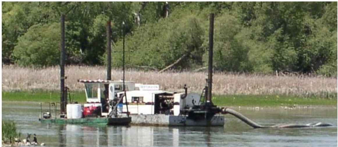
Figure 4. Dredge on Lake Faulkton.
