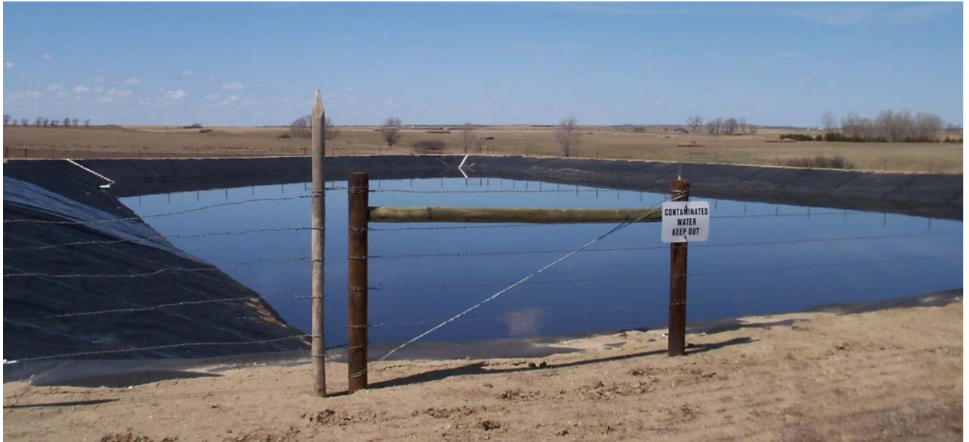
Figure 10: Animal Waste System Installed with Artificial Liner due to Light Soils.
