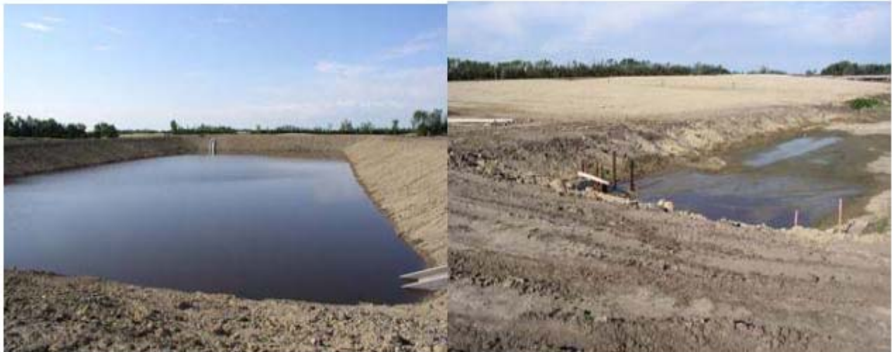
Liquid manure storage pond
