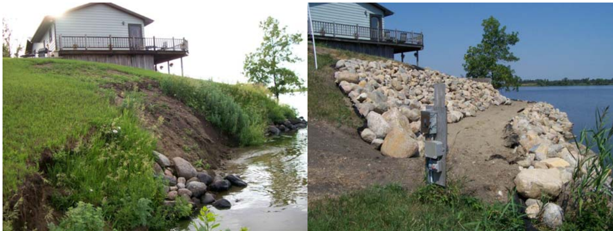
Figure 5. Mina Lake shoreline stabilized by reshaping and installing riprap.
