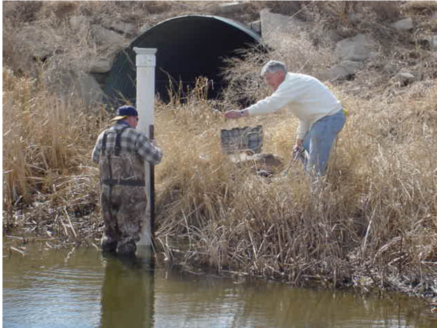
Figure 12. Installing a stage recorder at Rosette Lake.
