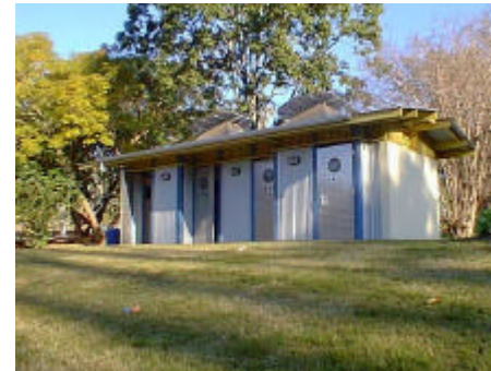
Photo 24 - the exterior of this public toilet is largely comprised of metal that is easy to clean.
