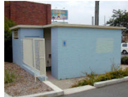
Photo 21 -an example of what can happen if there are not standard colours for public buildings. In this case, three (3) different light blue paints have been applied, and the patch to cover the graffiti is obvious.
