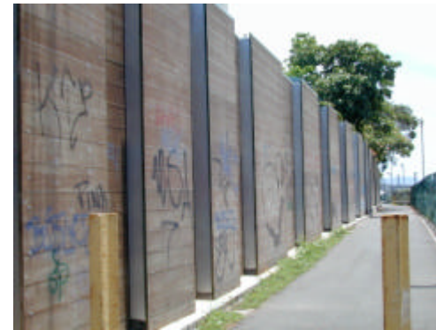
Photo 27 – untreated wood should be avoided. If it is required some form of treatment is necessary.
