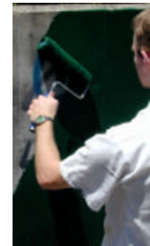
Photo 19 - in this case, a heavily tagged light-coloured concrete wall has been coated with dark green paint to enable easy graffiti masking.
