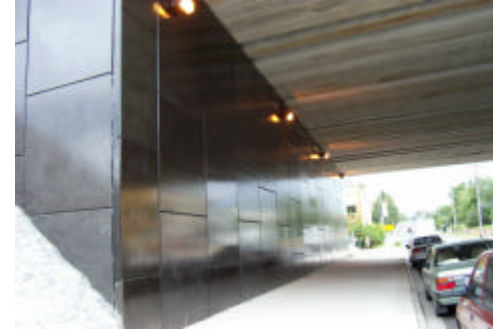
Photo 25 - an example of a likely graffiti canvas at a new development - a protective coating has been applied as a precaution
