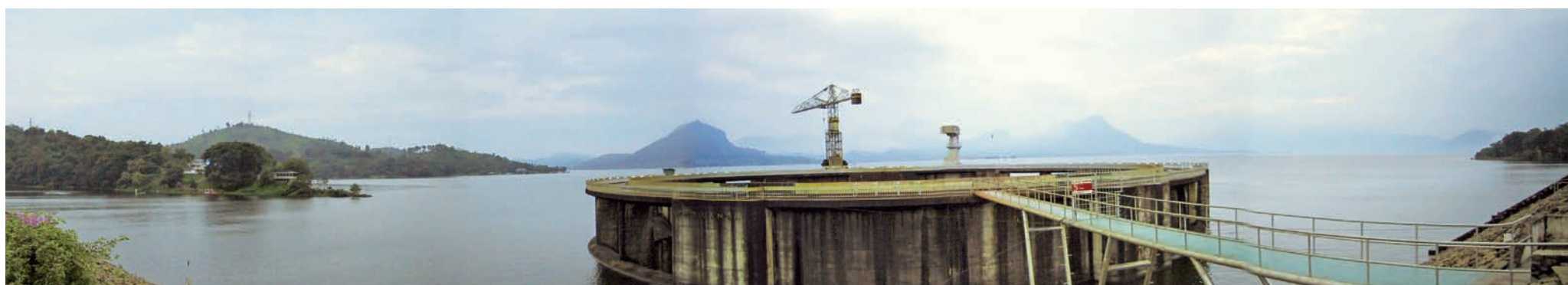
The journey that ends in your bucket. From left: Much of Jakarta's water gets its start in the Jati Luhur reservoir, before flowing into the trash-clogged Citarum River, where riverside toilets are a common sight. The water
