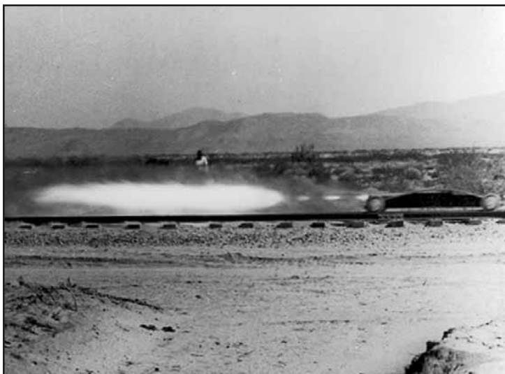
Top: An early wheeled rocket sled during tests on the Transonic (B-4) Track, 1948; China Lake was a pioneer in the design and operation of high-speed test tracks, operating several facilities over its more than 50 years in support of a wide variety of research, ordnance, and aircrew-safety programs.
