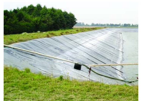
JE Piccaver & Co, based near Holbeach, grow baby leaf salads and rely on stored mains water for irrigation because the groundwater is too saline
