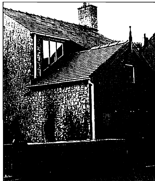
Conversion of joiner's shop to dwelling. Tideswell.
