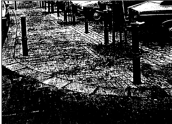
Concrete block paving with stone curbs and sets. Steel bollards of traditional design.
