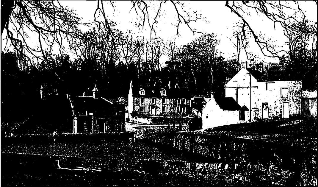
Open village with buildings well-spread allowing views of Monyash surrounding countryside: a feeling of spaciousness.
