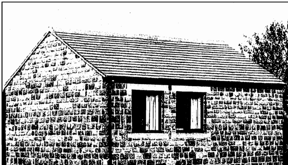
Simple cement-pointed verge and slightly projecting eaves on modern house.
