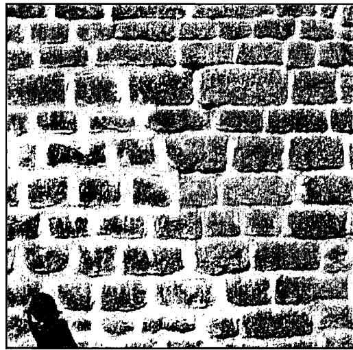
Bad pointing . . . joints too thick.
