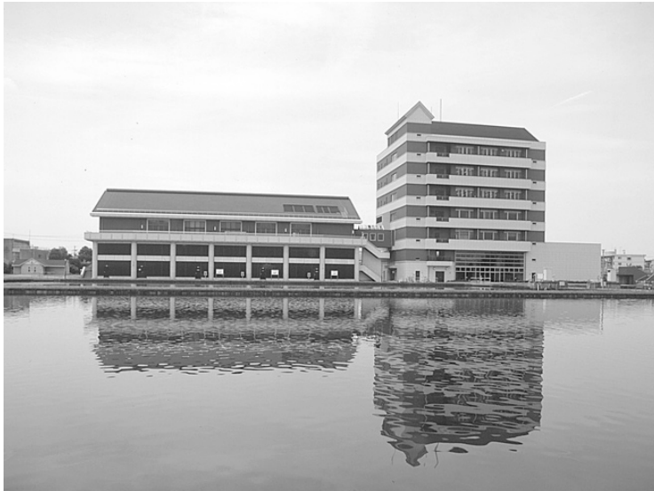
The Bureau of Waterworks. (Aichi Prefecture)
