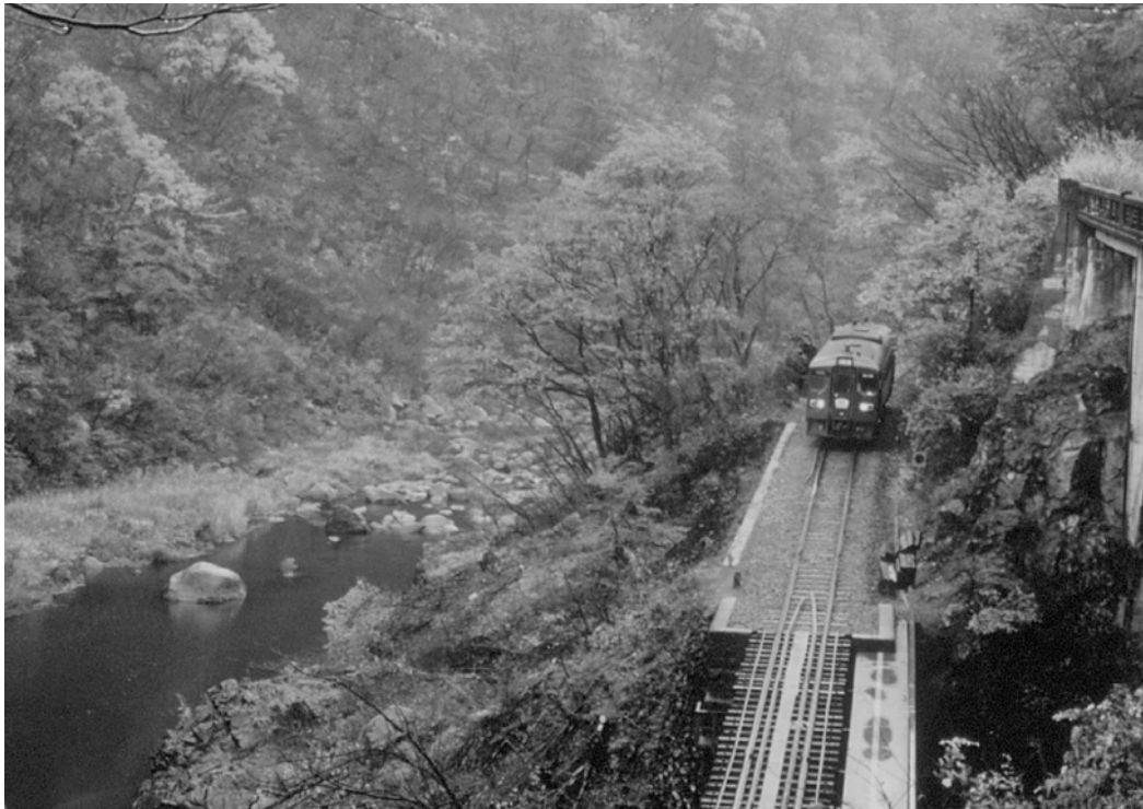
The 44.1-kilometer Watarase Canyon Railroad, built with third sector (combined government-private sector) funding. (Gunma Prefecture)
