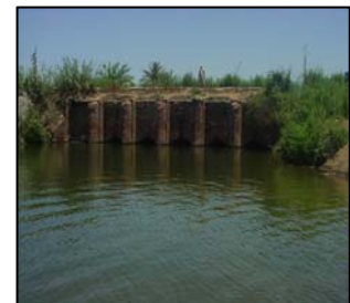
Picture (7-27) Hawis (to control water flow)
