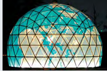
Center for Spirituality & Sustainability on SIUE campus. Geodesic dome designed by R. Buckminster Fuller
