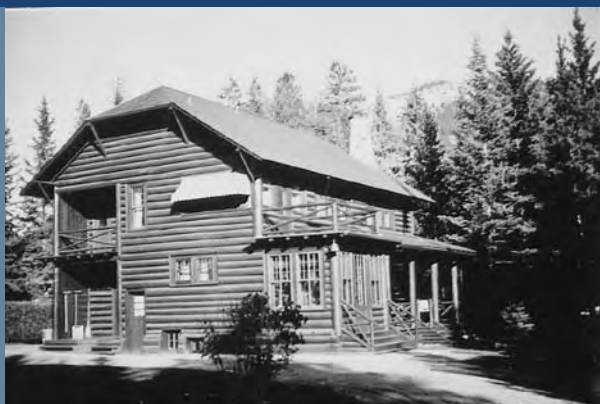
The Park Superintendent's residence on Buffalo Street, built in 1920 - 1937 Block B Lot 3-5
