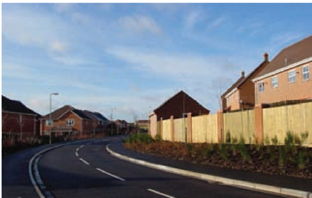
Road layout cutting off and dividing communities
