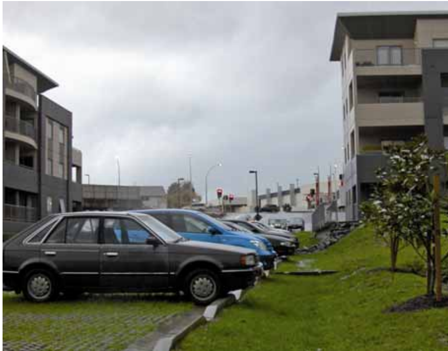
Figure 27: Permeable car park with discrete concrete blocks and mown grass between. Stormwater from the parking area runs into a grassed swale (centre). Photo: Robyn Simcock
