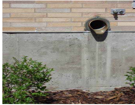
Figure 42 (a) and (b): Raingardens with minimal ponding depth in downtown Minneapolis, Minnesota, USA – right is the outlet to the downpipe – in this case a deep bark mulch replaces the more usual and longer lasting stones underneath the discharge point. Photo: Robyn Simcock
