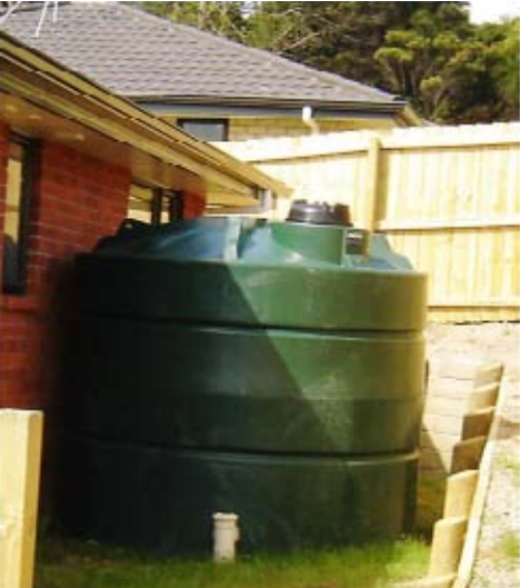
Figure 24 (a) and (b): Rain barrel and rain tank serve private houses. Left: The Netherlands, Photo: Marjorie van Roon. Right: North Shore City, New Zealand Photo: Penny Lysnar.
