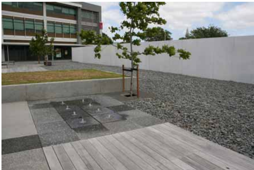
Figure 28: Courtyard with four different permeable surfaces: wooden decking, gravel, permeable pebble pavers (around tree) and grass, at Waitakere Civic Centre, Auckland, New Zealand. Photo: Maria Ignatieva
