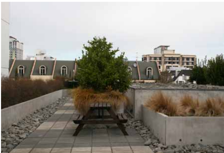
Figure 22: Intensive green roof, Environment Canterbury, Christchurch, New Zealand. Photo: Maria Ignatieva
