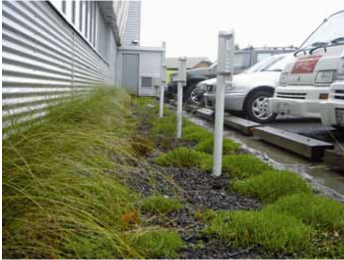
Figure 35: Bioretention swale, Landcare Research, Auckland, uses Carex against the building with low groundcovers Selliera radicans, Pratia angulata, and Acaena microphylla. Raised wooden barriers allow unimpeded (sheet flow) runoff into the swale while excluding vehicles. Photo: Robyn Simcock
