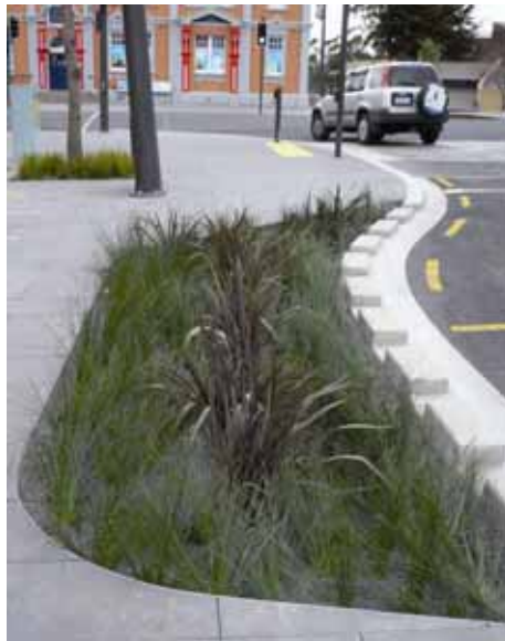
Figure 40: Hunt Street (Hamilton) raingardens have a fine gravel mulch; water enters from the road through slots in the curb (Megan Wraight – Wraight and Associates Landscape Architects). Photo: Robyn Simcock
