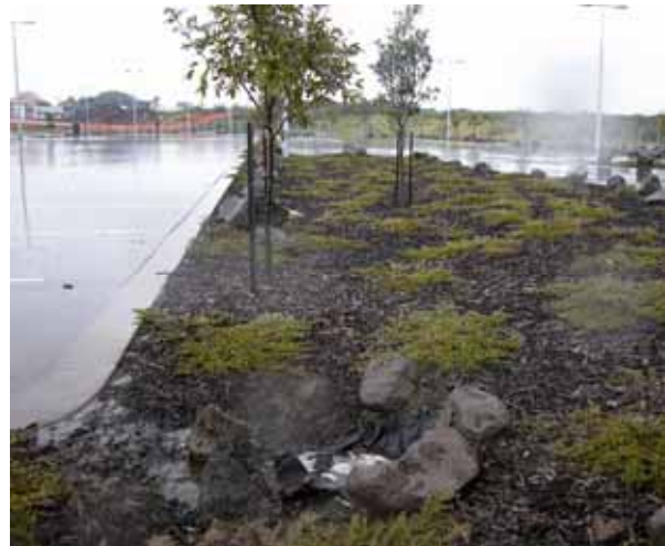
Figure 34: Swale, Auckland Netball Centre car park, with prostrate coprosma groundcover. Boulders deter cars from trafficking over the swale and have also been placed around the grate that pipes overflow to a pond – to disrupt the water flow. Photo: Robyn Simcock
