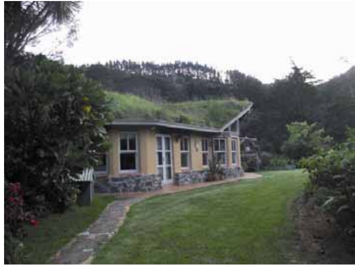
Figure 19: Extensive green roof on a private house in Matakana north of Auckland, New Zealand. Photo: Marjorie van Roon
