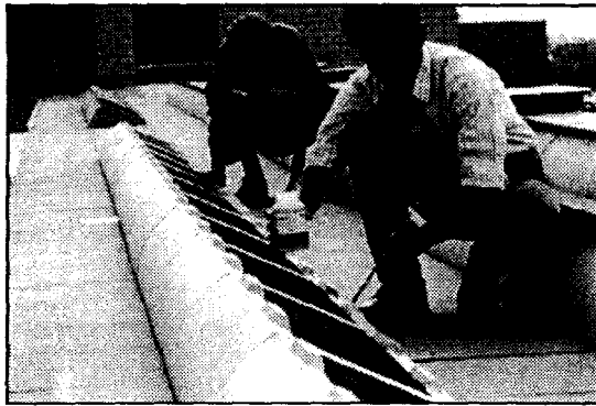
Figure 19.7 Flat roof installation: Cleaning and priming of concrete block
