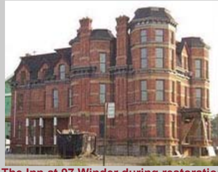
The Inn at 97 Winder during restoration
