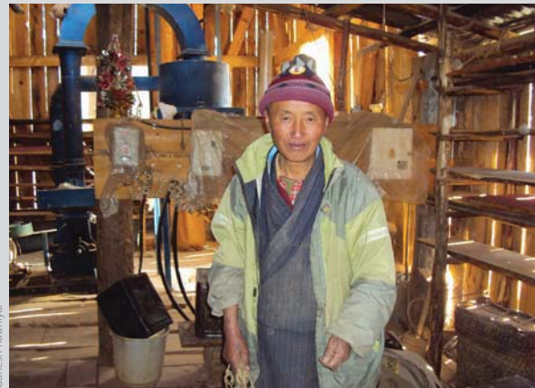
Empowered: newly installed equipment in a Bhutan rural business
