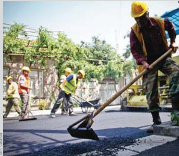
ADB has supported infrastructure upgrades in Adigeni
