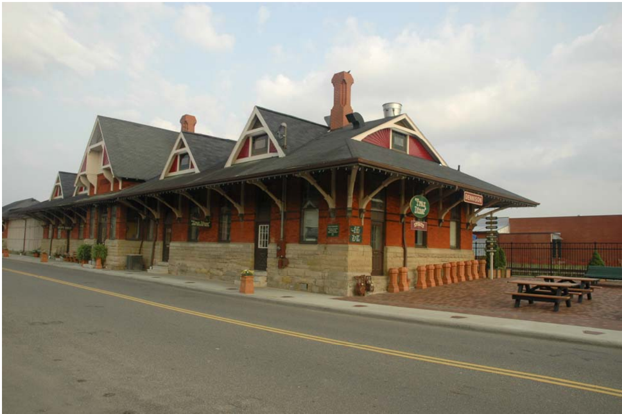
PENNSYLVANIA RAILROAD DEPOT AND BAGGAGE ROOM, DENNISON, OHIO (NHL, JUNE 17, 2011)
