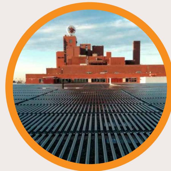
A view from the roof of the Newark Brewery, which installed a solar array of more than 7,000 photovoltaic solar panels. At peak production, solar power will be capable of covering nearly 10 percent of the brewery's electricity demand.
