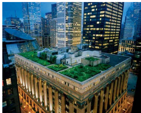
Green Roof on top of City Hall in Chicago Photo by Diane Cook and Len Jenschel (National Geographic)
